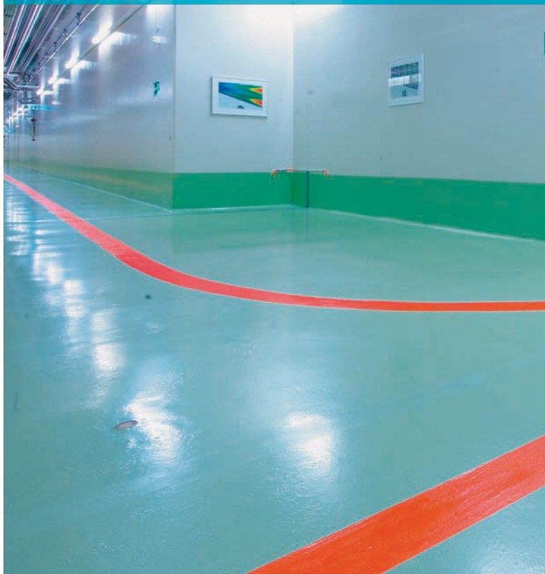
TRANSPORT TUNNEL BETWEEN CONDITIONING PLANT AND STORAGE BUILDINGS
